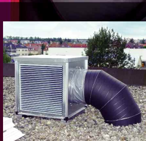
Roof installation with outdoor cover hood rain repellent grille (accessories).
